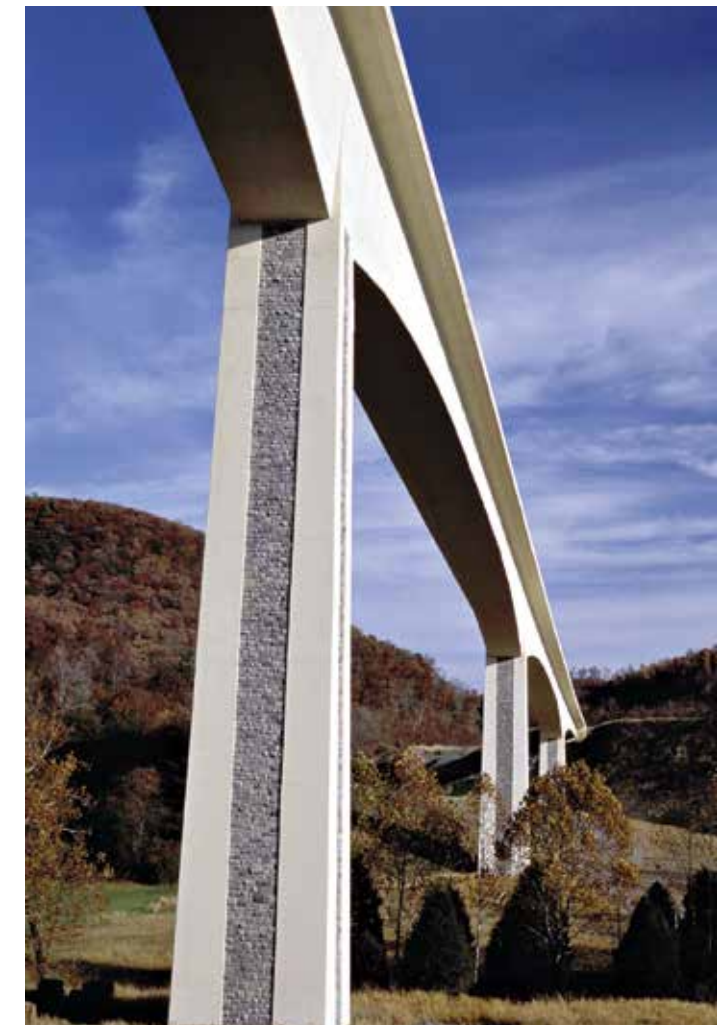
Smart Road Bridge
