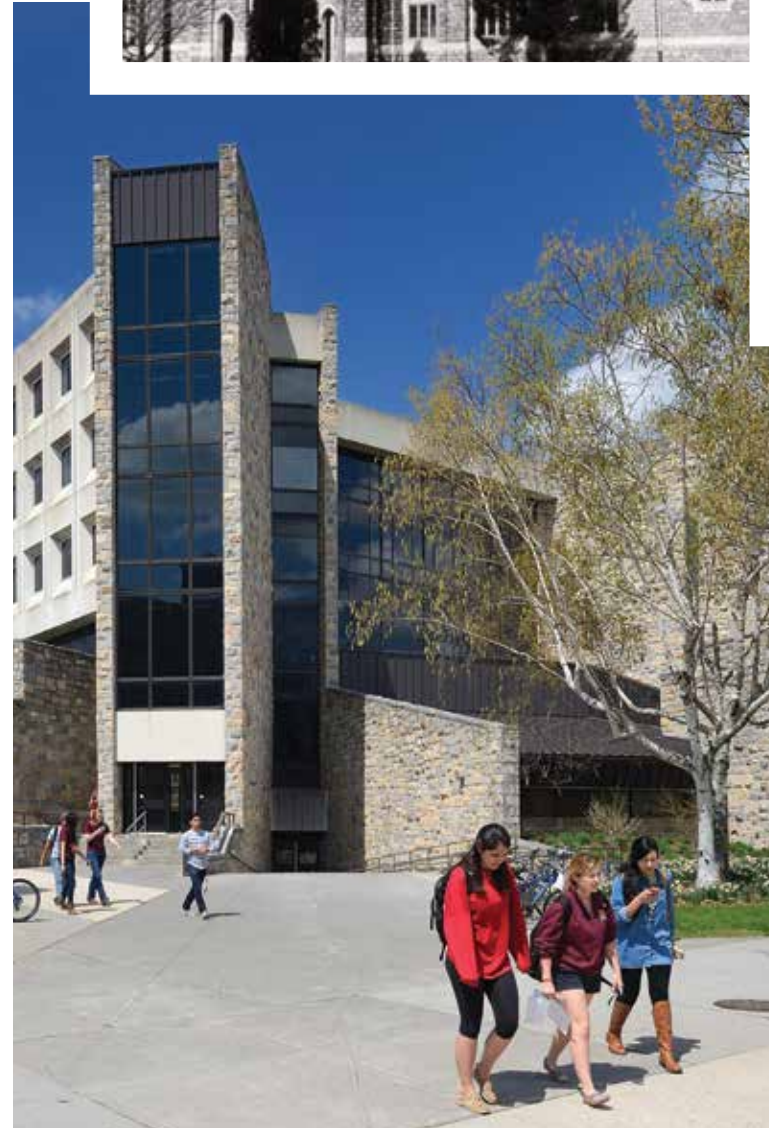
The original McBryde Building of Mechanical Arts (top) combined Hokie Stone with the neo-Gothic architectural style. The newer McBryde (above) was completed in 1971.
